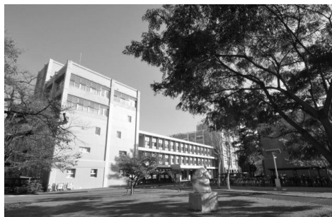
Building of the Cooperative Faculty of Education
