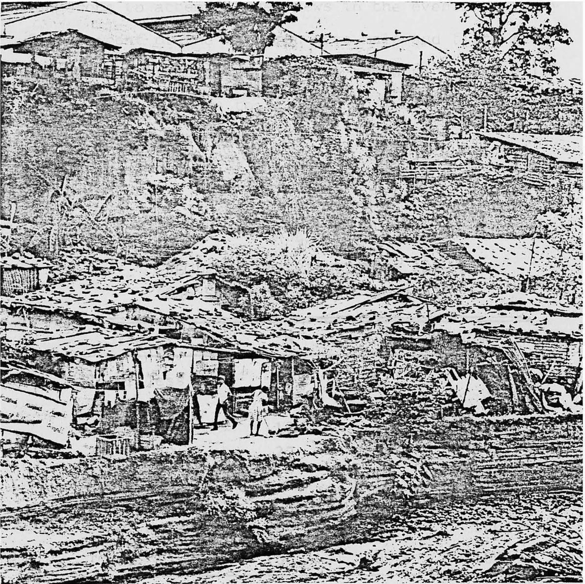
Figure 10. Typical Shacks in a Shanty Town.
